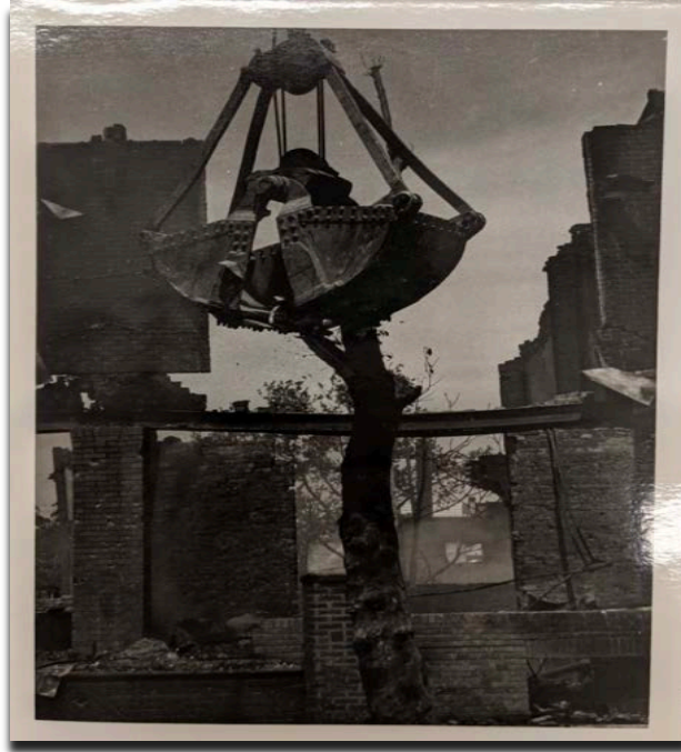
The clamshell crane bucket being used to excavate the MOVE remains from 6221 Osage Avenue
